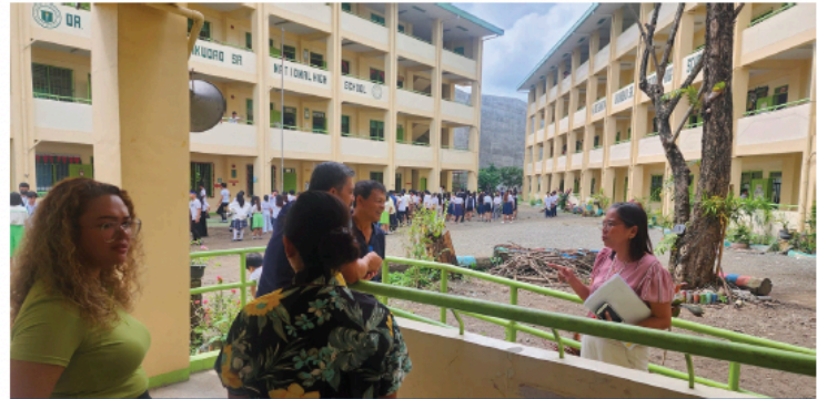
Site inspection for future project; concreting of flag raising area, to be sponsored by Rotary Club of Lahaina Hawaii
