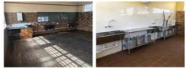
The kitchen at Mary Waters High School before (left) and after (right) renovation Photos by Gavin Keeton
